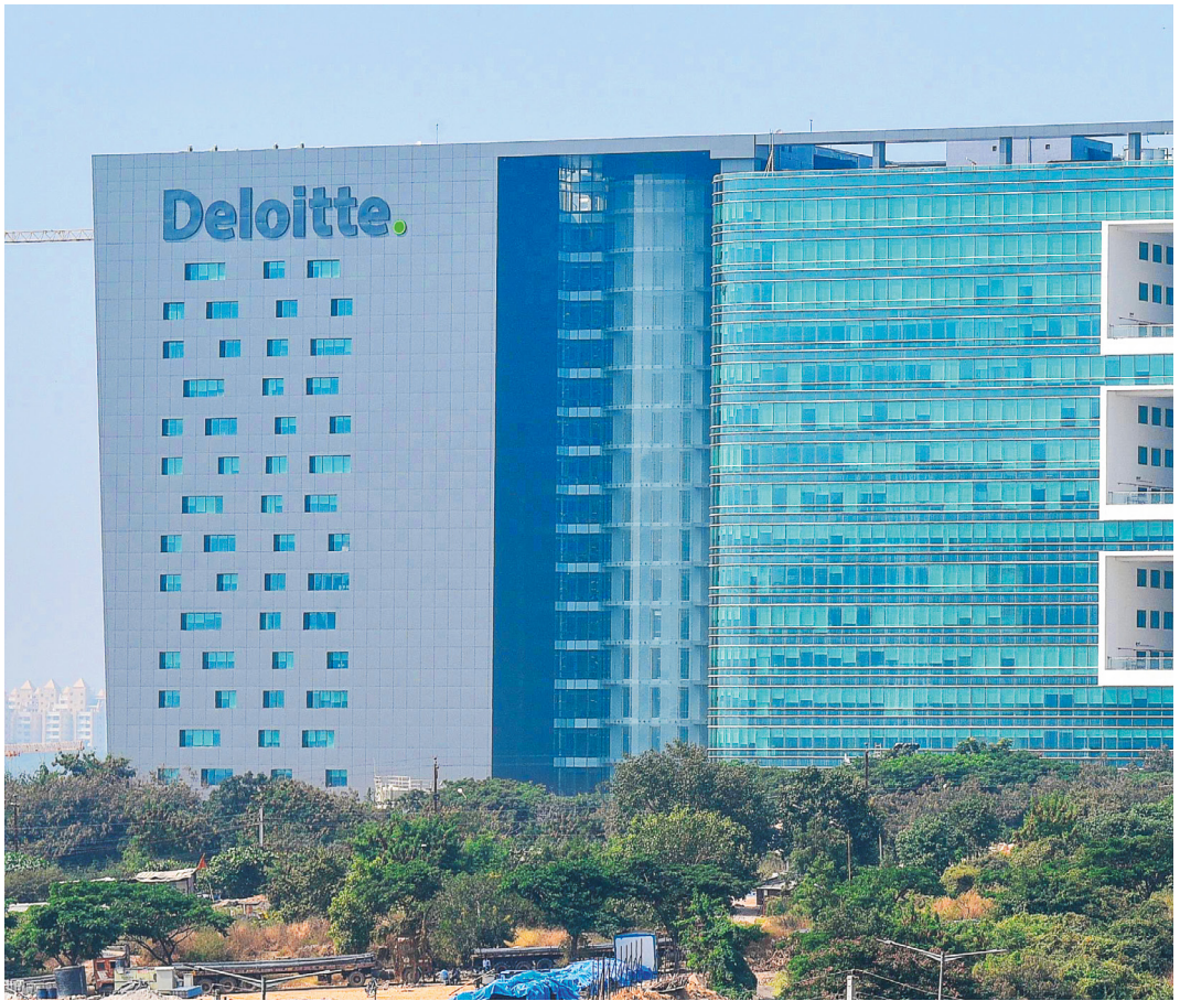
Deloitte's office building in Hyderabad, India. Its glazed facade required 76% less installation time than brick exterior walls.
