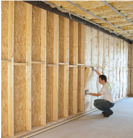
Up to 80% of the energy needed for heating or cooling can be saved by insulating. Here, an interior insulation project. © Isover
